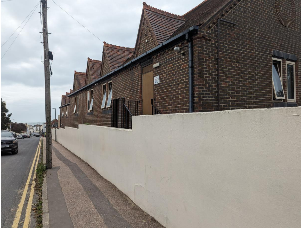
Boundary wall between Brighton College and Walpole Road
